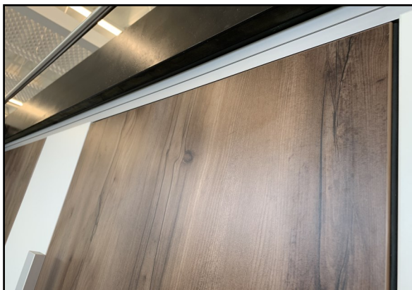
Floating configuration with recessed pedestal and headrail and shadow gap wall connection
